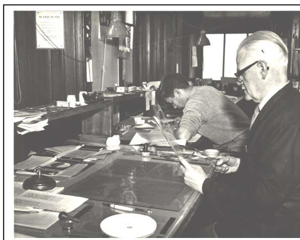
Above: Bartholomew staff patching plates with lithographic film
